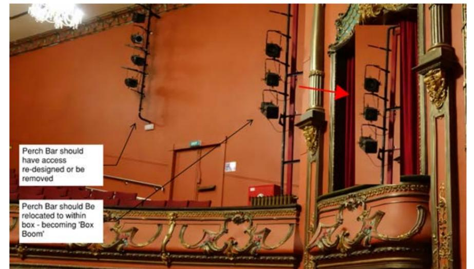
Figure 3: Perch bar redesign requirements
