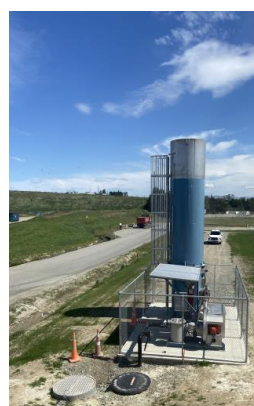
Redruth Landfill Cell 3.5 and Gas Flare
