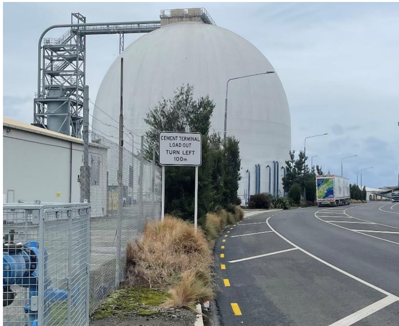
Photo 2 Holcim Cement Terminal advance warning sign.
