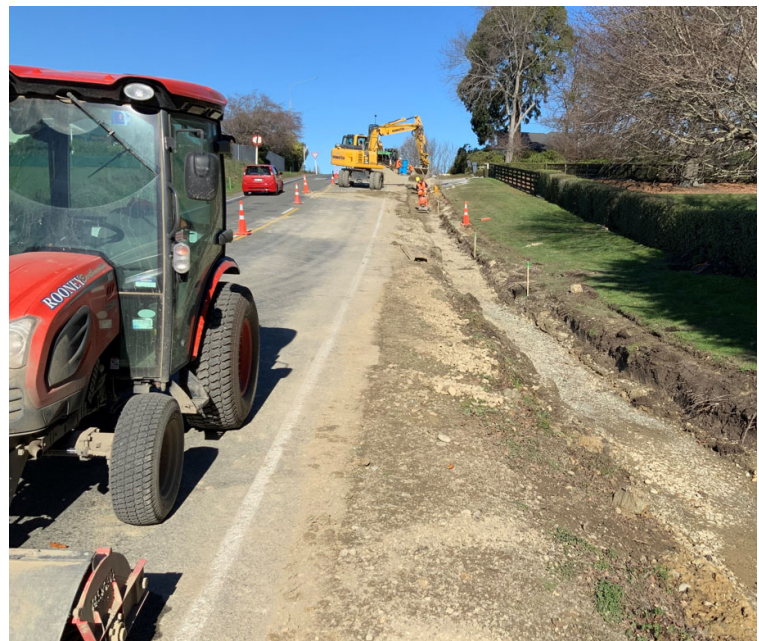
Washdyke Water Network Improvement Stage 1.
