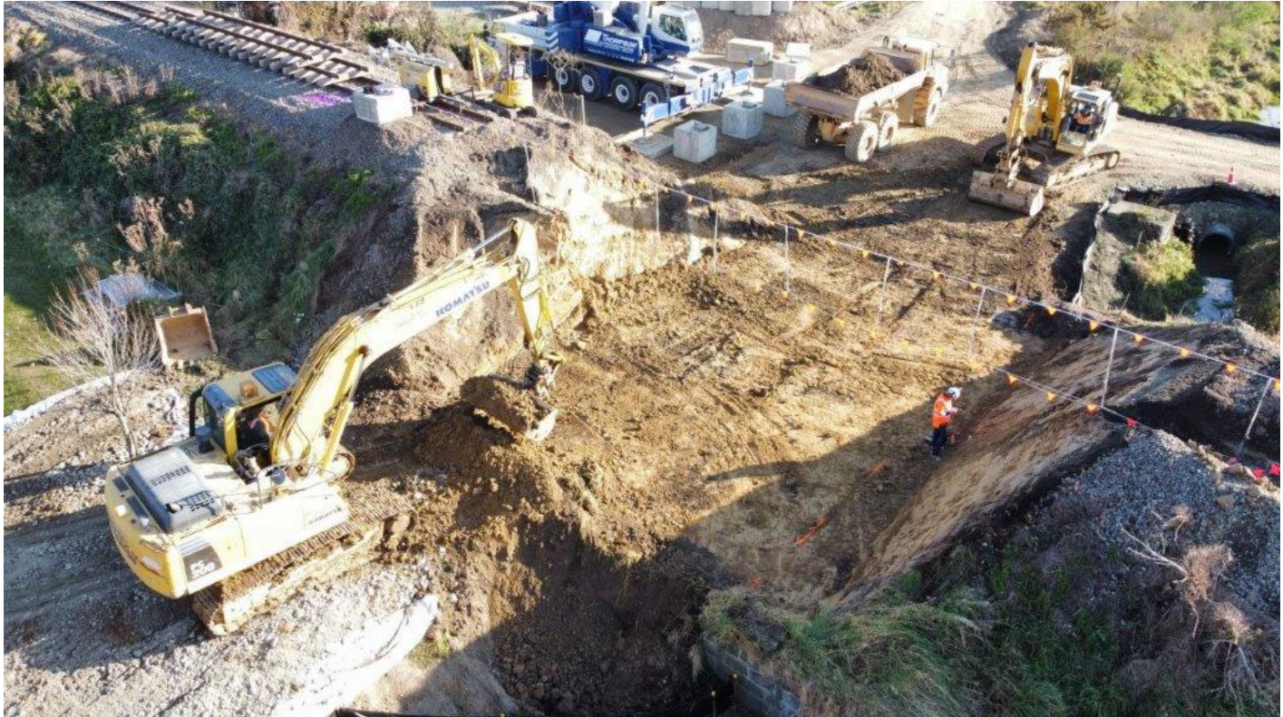
Taitarakahi Creek new culverts under construction.
