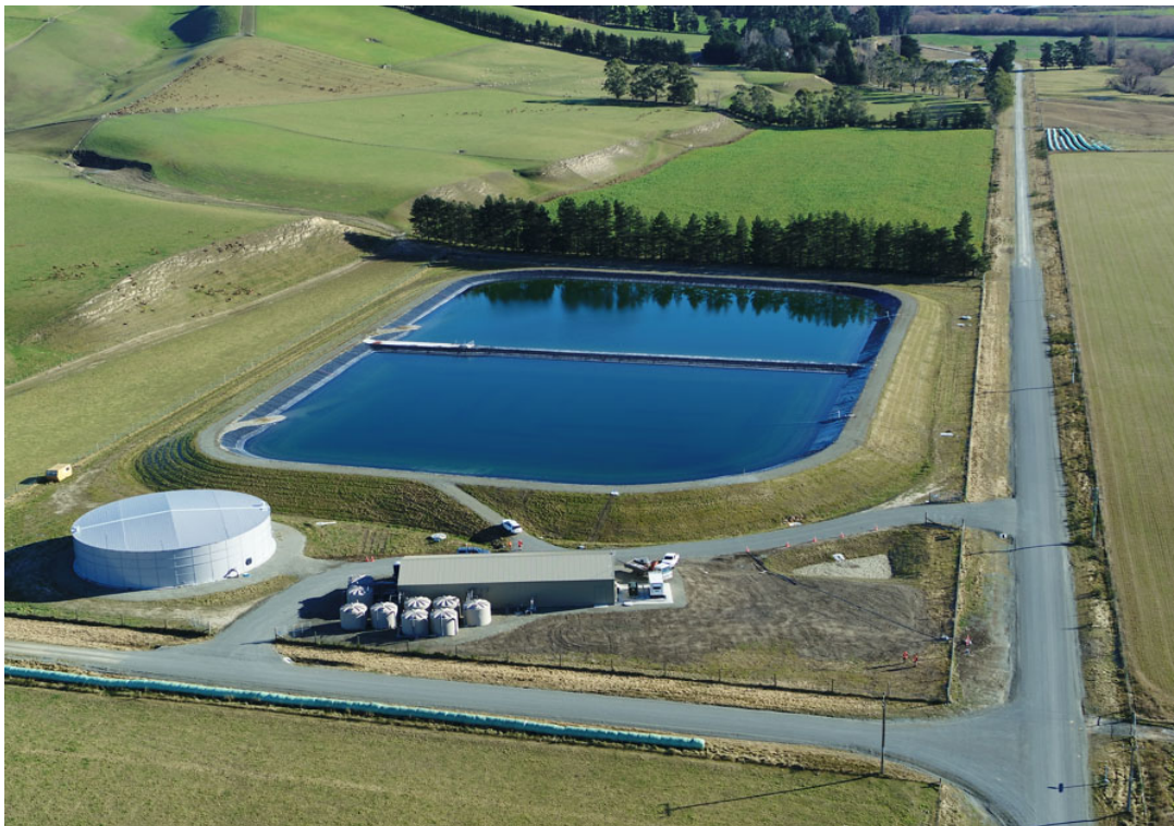
Drone photo of Te Ana Wai Water Treatment Plant, Treated Water Reservoir and Raw Water Storage Ponds.
