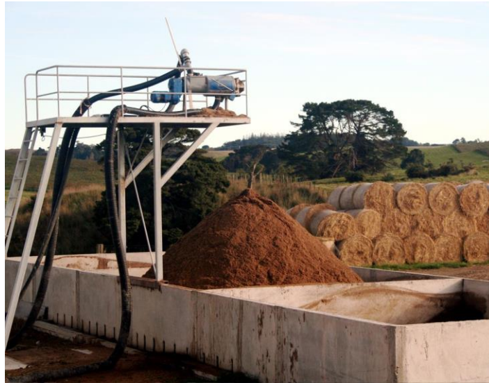
Photo 7: Screw press type of solids separator
