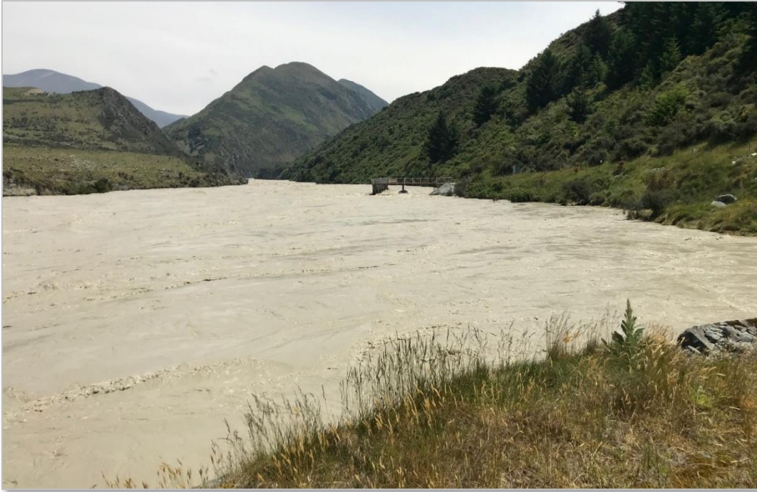
Fig 3 View of the Rangitata River in flood (Dec 2009). The rock weir is fully submerged and approximately 65% of the weir was eroded by this event.
