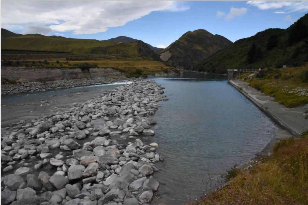
Fig 2 This photo is taken at river level looking out across the rock weir. The intake structure is on the right of the picture. The level control function of the weir is evident – the water level behind the weir is higher than below it – and the navigable gap can be seen towards the far side of the weir. In this illustration, the weir has been recently maintained.
