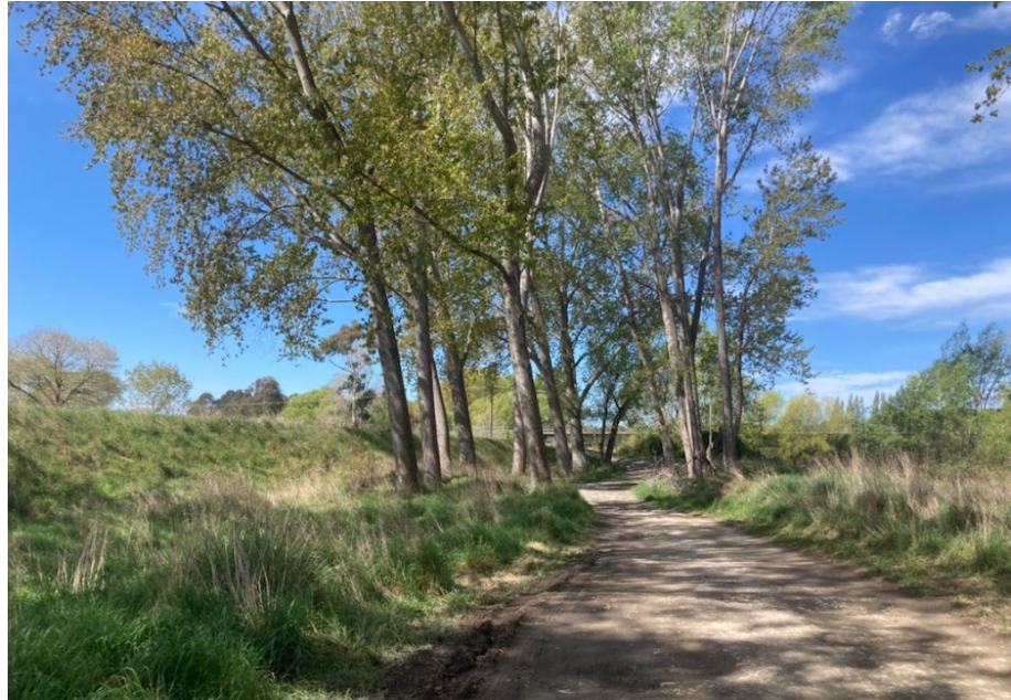
Figure 3: Current large trees that pose a risk to a stopbank (left) and access (centre-right).
