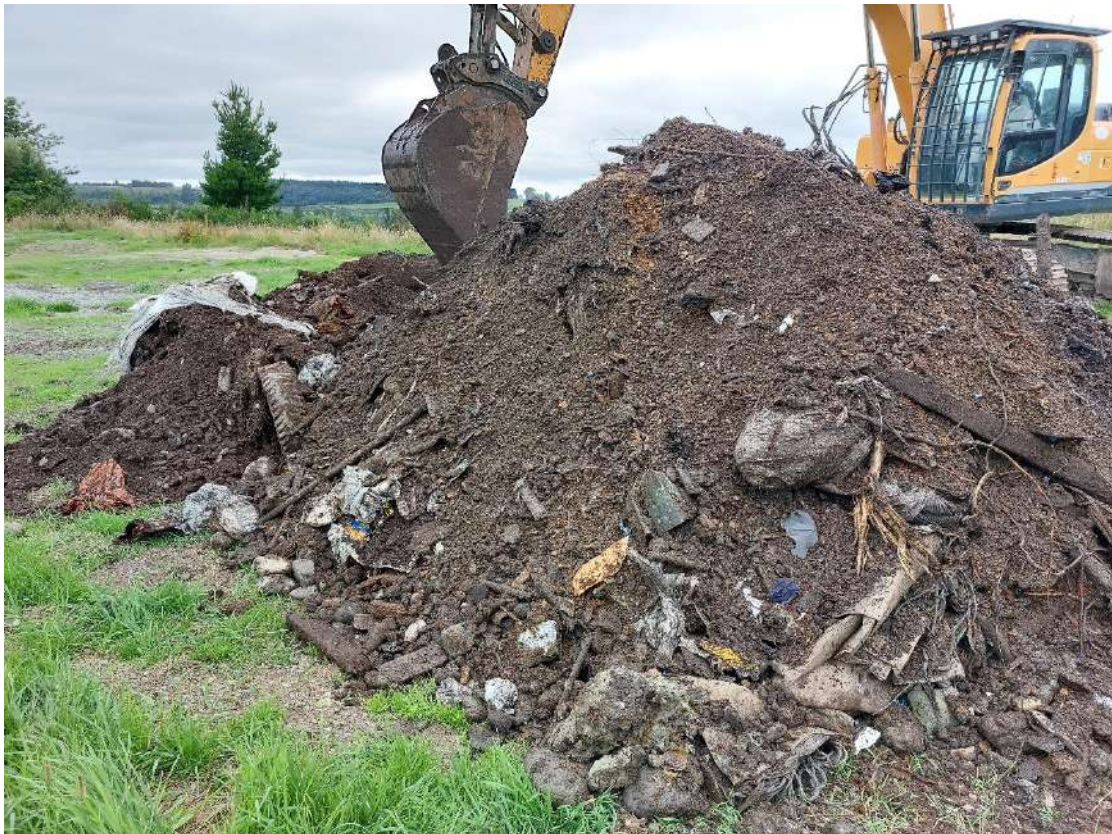
Photograph 8: TP101 arisings (before screening)
