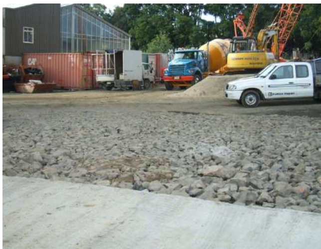
Stabilised entranceway (Source: SouthernSkies)
