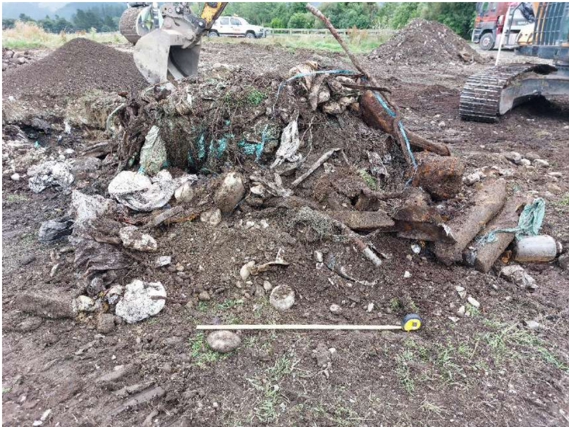
Photograph 40: TP107 coarse arisings that were separated out by the excavator bucket.
