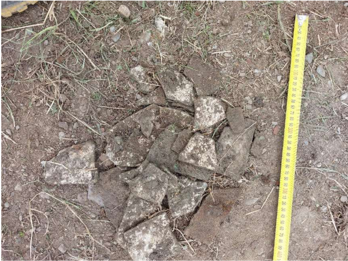
Photograph 19: ACM fragments separated from TP103 arisings.
