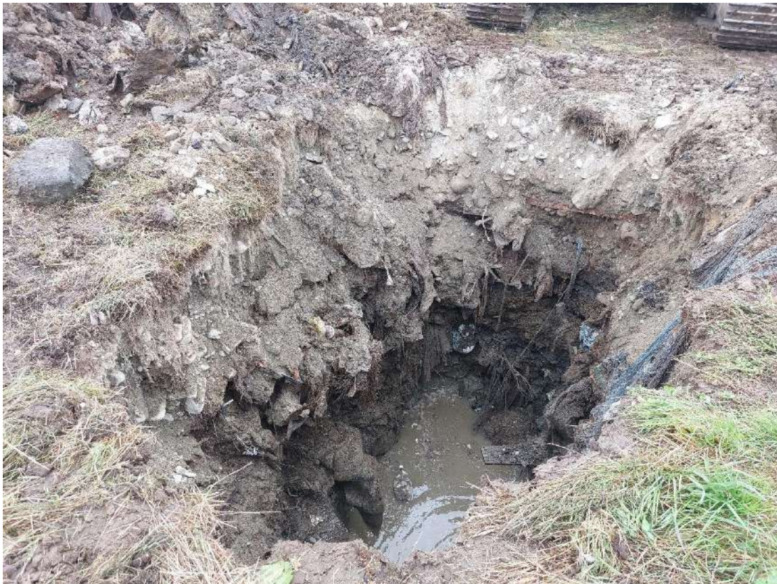
Photograph 24: TP104 excavation. Perched groundwater can be seen at the base.
