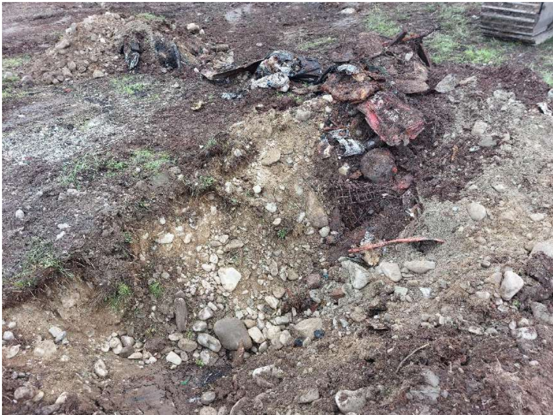
Photograph 38: TP107 'Cover' material and underlying 'Waste Mix'.
