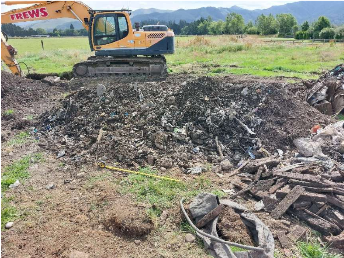
Photograph 11: TP101 Stockpile of material which did not pass through the 25 mm screen.
