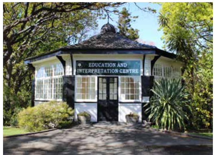
Timaru Botanic Gardens Education and Interpretive Centre building was modernised, including interior and exterior painting.
