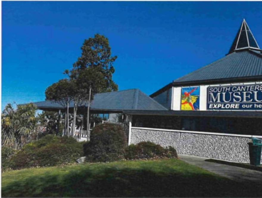
North/East elevation - Main entrance
