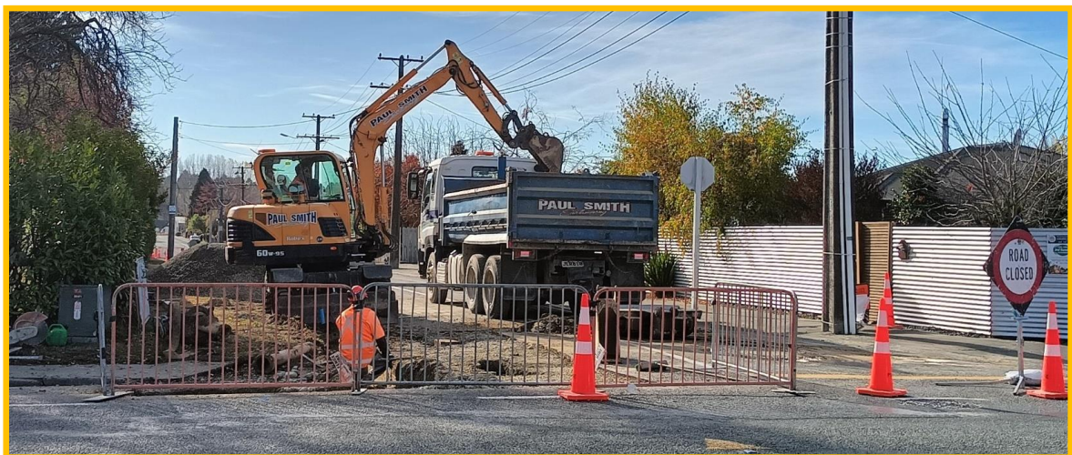
Construction in Progress – George Street, May 2024
