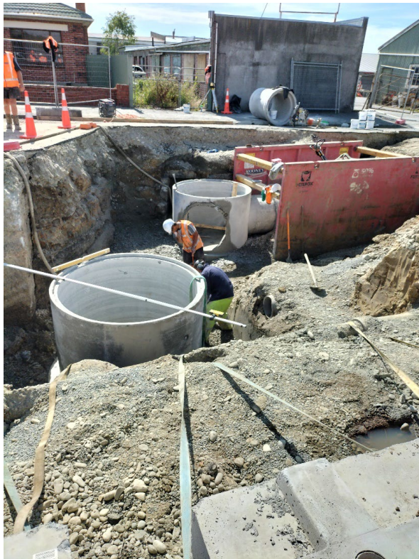
High St Stormwater Main
