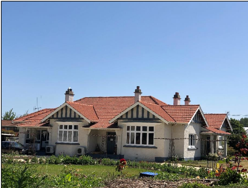
Former vicarage of St Peter's Church at 199 King Street.
