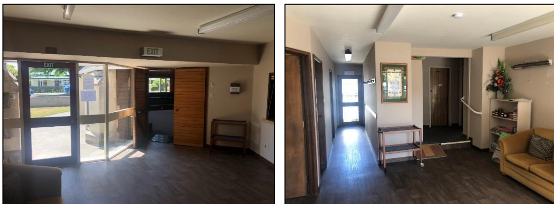
Left: View of entrance lobby from vestibule. Right View of corridor at left leading to south toilet entrance at end, and vestibule leading to north toilet and vestry to the right of the image. Source: DPA Architects. January 2020.
