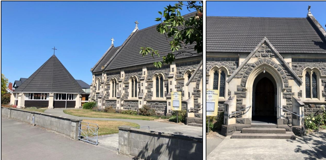
Left: North elevation of church with 1978 octagonal Parish hall at eastern end. Right: entry porch to nave. Source: DPA Architects, January 2020.
