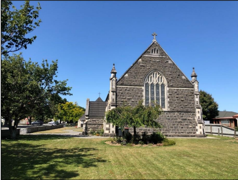
West elevation of church facing King Street. Source: DPA Architects, January 2020.
