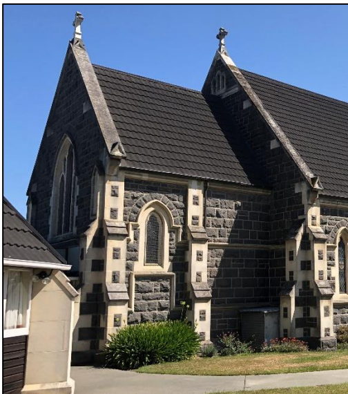
St Peter's eastern gables. Source: DPA Architects, January 2020.
