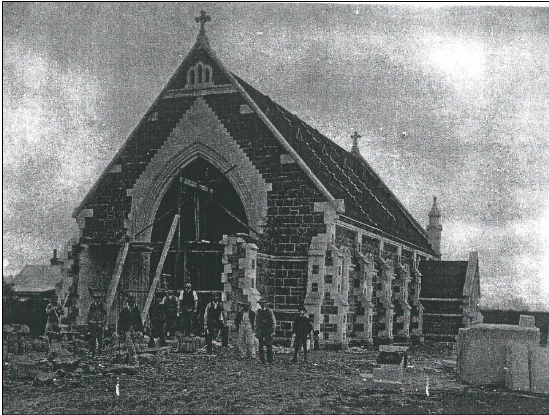
View of St Peter's Church under construction. John Langridge is pictured with walking stick alongside other working men, all of whom stand in front of the chancel arch at the east end of the church. Source: Sheila Langridge, From Sussex to Canterbury: the story of the Langridge family , 1999, p33.
