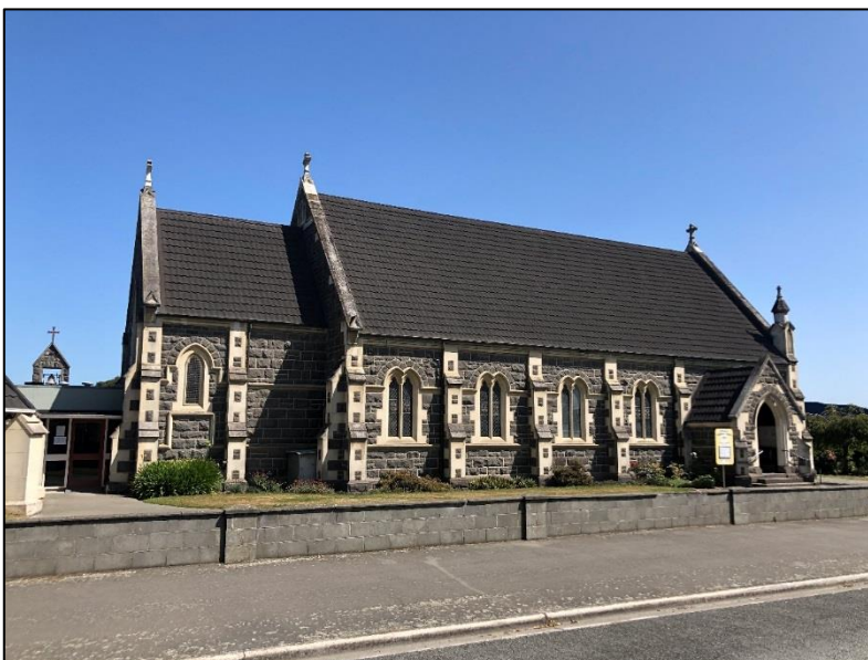
North elevation of church facing Dyson Street showing the gabled entry porch to the western end and the chancel with a lowered roof line to the eastern end. Source: DPA Architects, January 2020.
