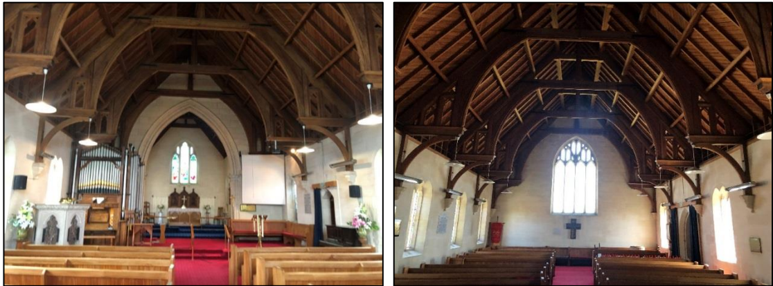
Left: View east down aisle of nave toward the chancel. Right: View west from the chancel toward the rear wall of the church facing King Street. Source: DPA Architects, January 2020.
