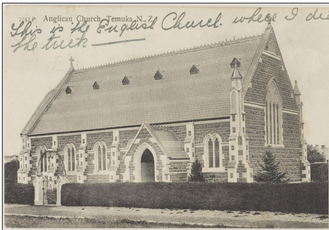
1907 postcard of St Peter's Church, Temuka. Note the original concrete Gothic posts and steel gate, now removed. Source: Muir & Moodie Studio.
