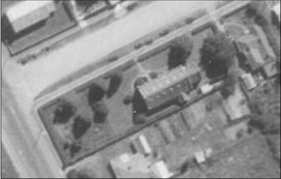
Aerial photograph 26 February 1939 showing original form of church with nave, chancel, entry porch to north elevation and sacristy to south elevation. The six dormer roof vents to the north and south roof planes of the nave are clearly visible. There appears to be an outbuilding to the south of the chancel. The image shows the early fencing treatment with hedging and numerous trees in the allotment. Source: Retrolens Historical Image Resource, SN86.
