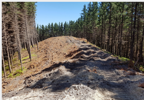
Road corridor after road-line salvage and prior to clearing and stripping.
