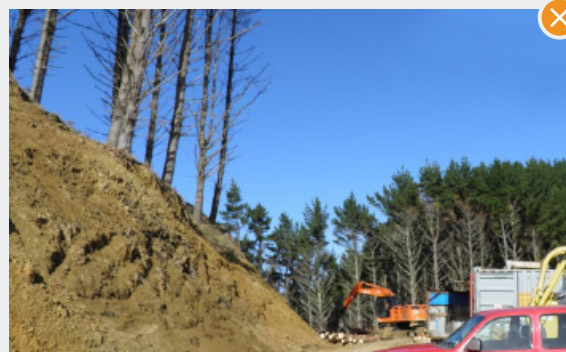
Trees left standing above a landing site present a significant hazard. This risk would have been eliminated if trees were removed during road-line salvage .
