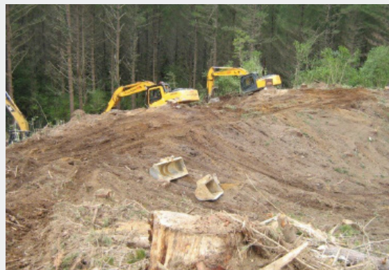
Excavators clearing vegetation and stripping topsoil ahead of landing construction.
