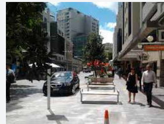
Fort Street Shared Street Auckland
