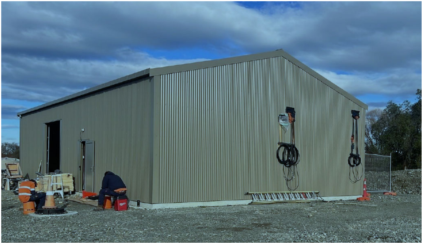
Exterior of Te Moana Water Treatment Plant
