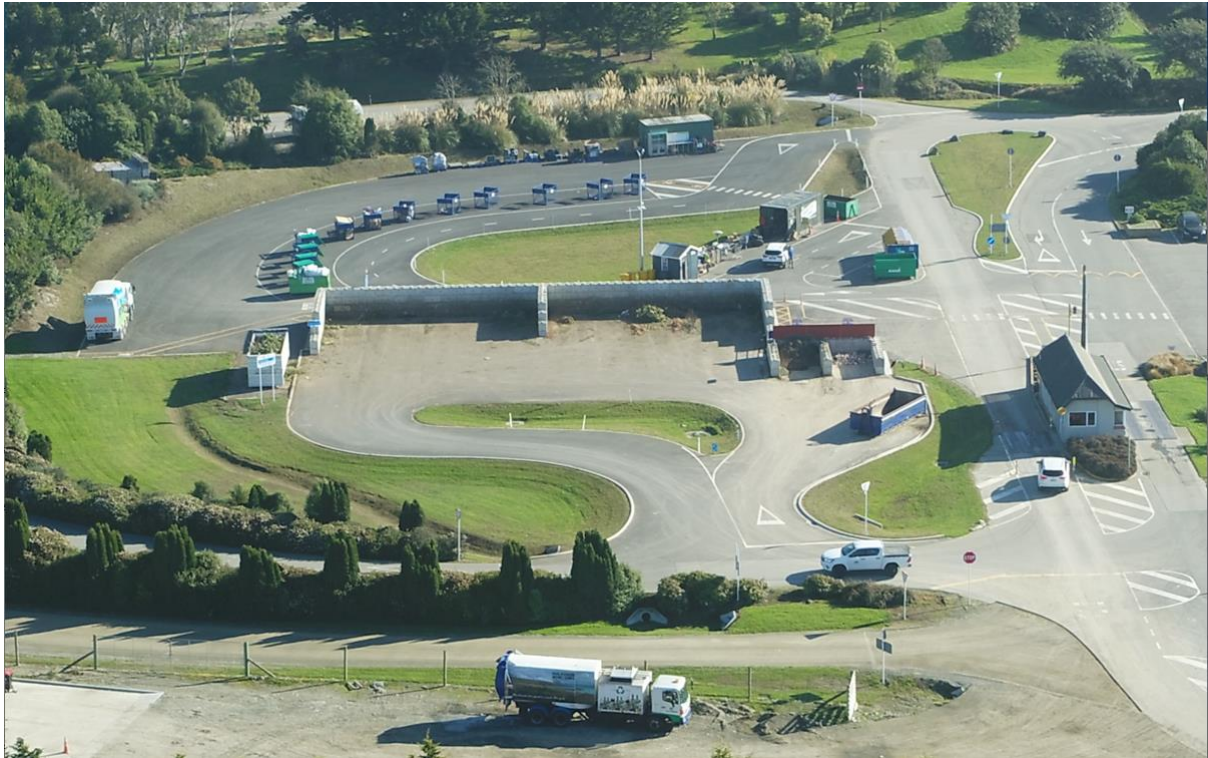
Figure 7 Image of Redruth Resource Recovery Park
