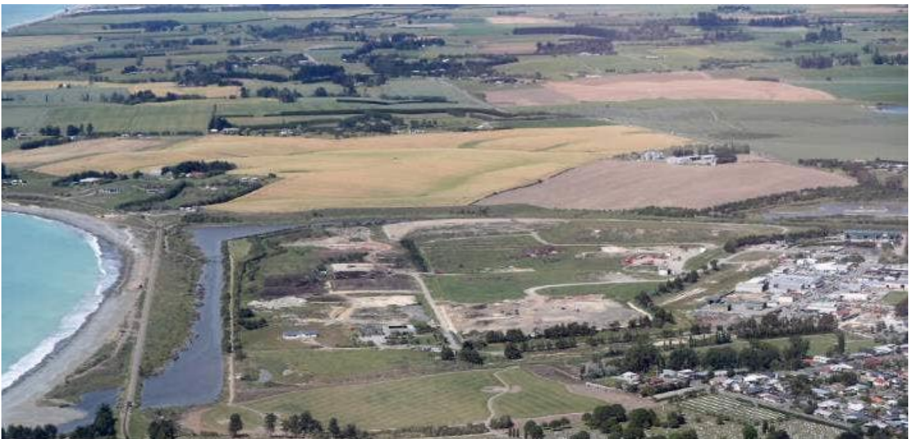
Figure 10 Image of the Redruth Facility
