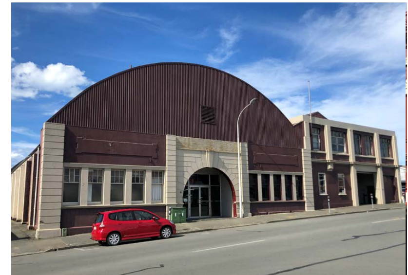
Former Olympia Hall and 1911 Garage.
